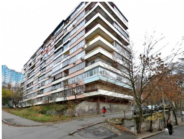
Fig.162. A typical 9-storey residential block with perimeter balconies (1970s)
