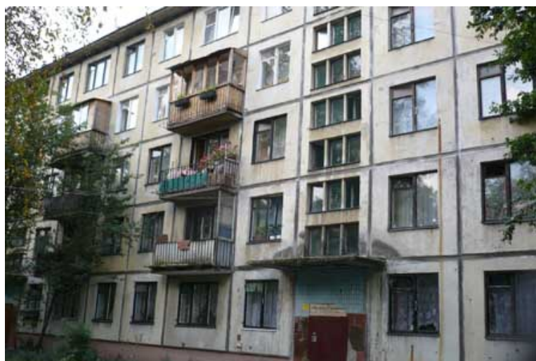
Fig.159. A typical 5-storey residential block made of ready-made concrete blocks.
