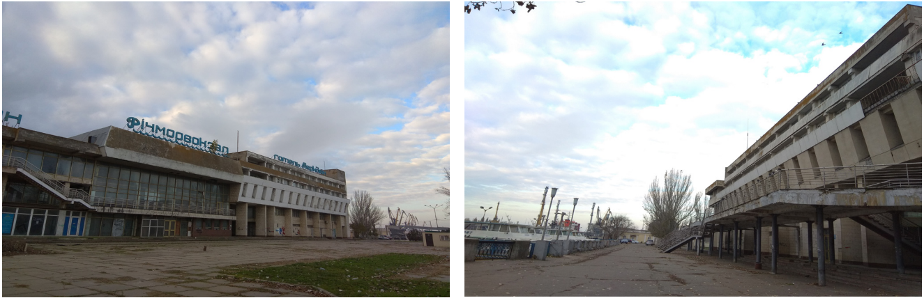
Fig. 2. The current state of the premises of "Richmorvokzal" and adjacent public spaces (Photo: D. Malchykova, 2020)
