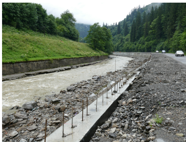
Photo 7. The channel on the section 22
