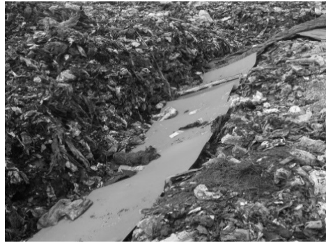
Fig. 3. Plastic sheets for side insulation
