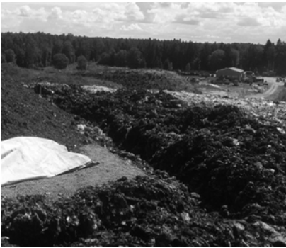
Fig. 2. Excavation of trenches
